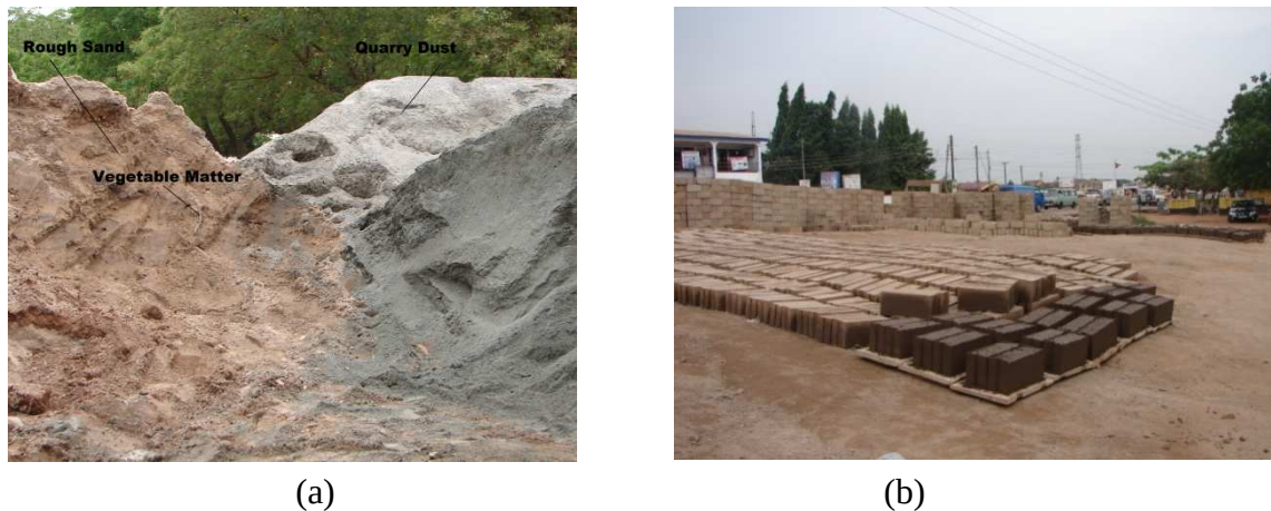
Fig. 2 (a) Rough Sand and Quarry Dust (b) Sandcrete Block work
