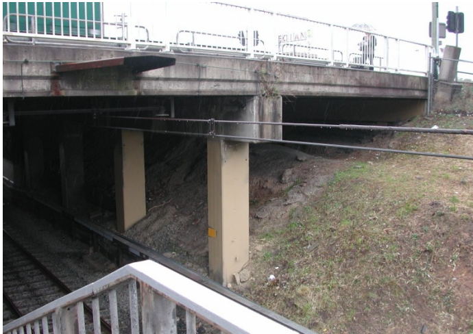
Figure 5: Views of northbound bridge prior to construction
