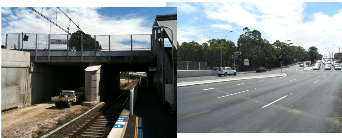
Figure 6: View of completed bridge from platform level and road level
