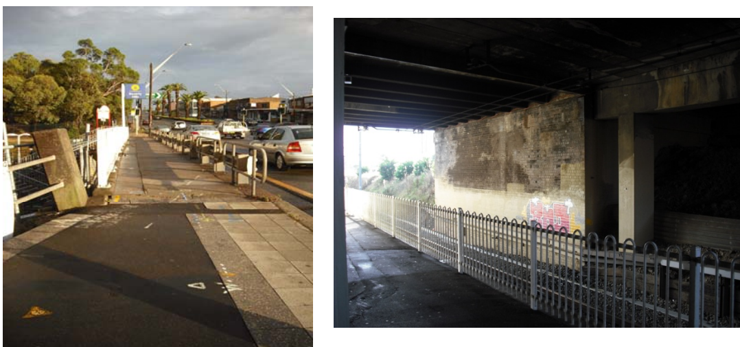
Figure 1: King Georges Road Overbridge – Views from on top and under bridge
