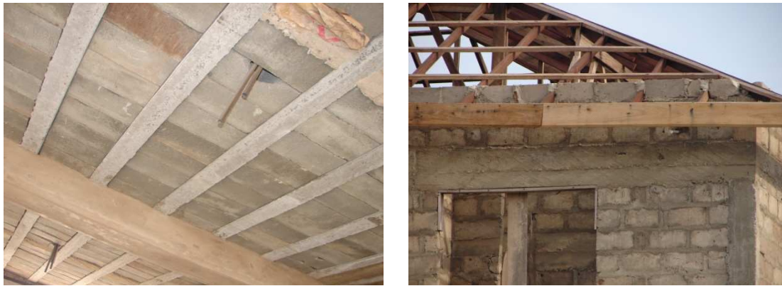
(a) Fig. 3 (a) Precast Floor Slab System
